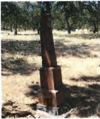
8a. Tilted granite obelisk at risk of falling.
