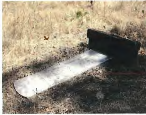
8b. Fallen marble tablet marker that can be easily repaired by resetting.
